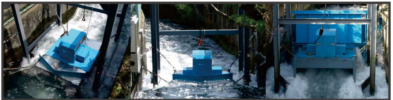
STREAM Unit installed in agricultural waterway, Tsuru City Yamanashi Prefecture
